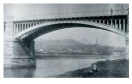
the masonry was examined, and found to be satisfactory. The viaduct began to show signs of subsidence some years after the line was opened (this was probably due to heavier axle-loads) and many of the piers had to be braced with iron tie-bars and flanges.
